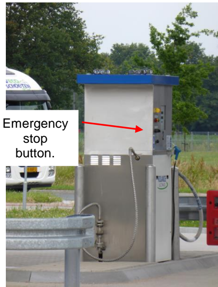
Supply point with emergency stop button.
