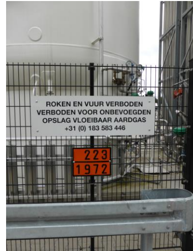
Recognisability of LNG &amp; contact details of the operator in the vicinity of the storage tank
